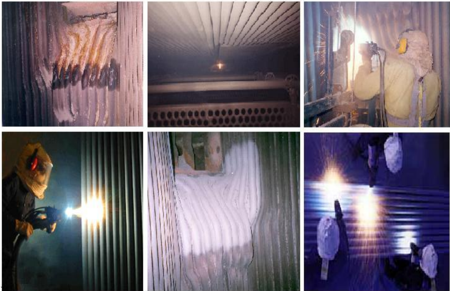
Boiler tube coating being done by IPM at site.
